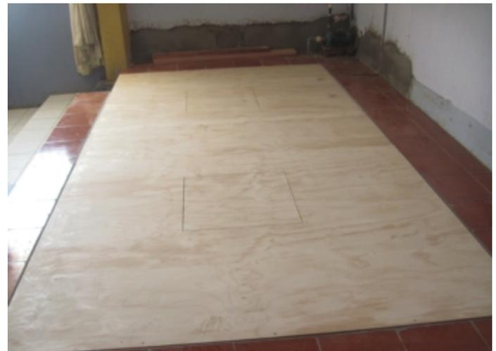
Following installation of the water storage tanks and plumbing, carpenters built a wooden support structure and cover so the area can continue to be used as a stage in the church’s chapel.
