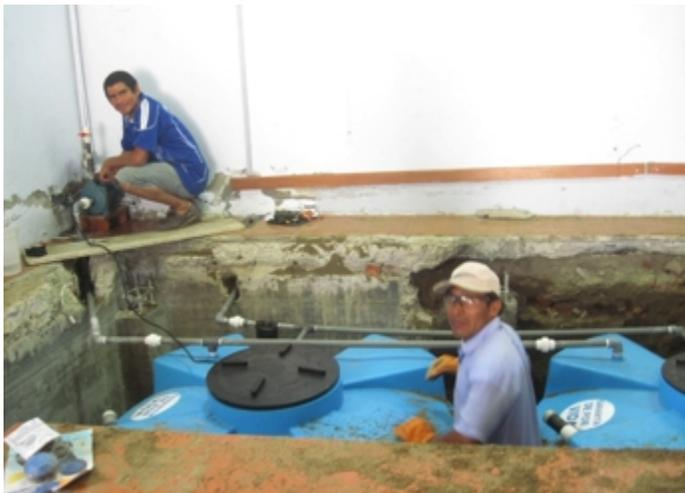
Professional installers check the operation of the water pump and look for leaks in the water storage tanks and new plumbing.
