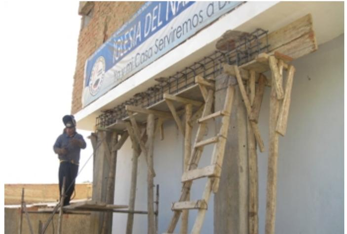
Reinforced pillars and girders were installed outside and inside the building to support the weight of a water reservoir installed above the kitchen area.
